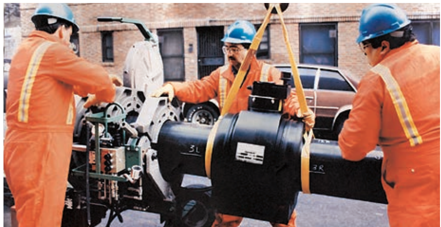
12" Poly-Gas® valve fusion operation
