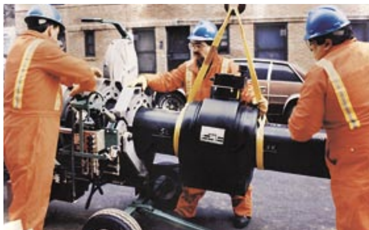
12" Poly-Gas ® valve installation
